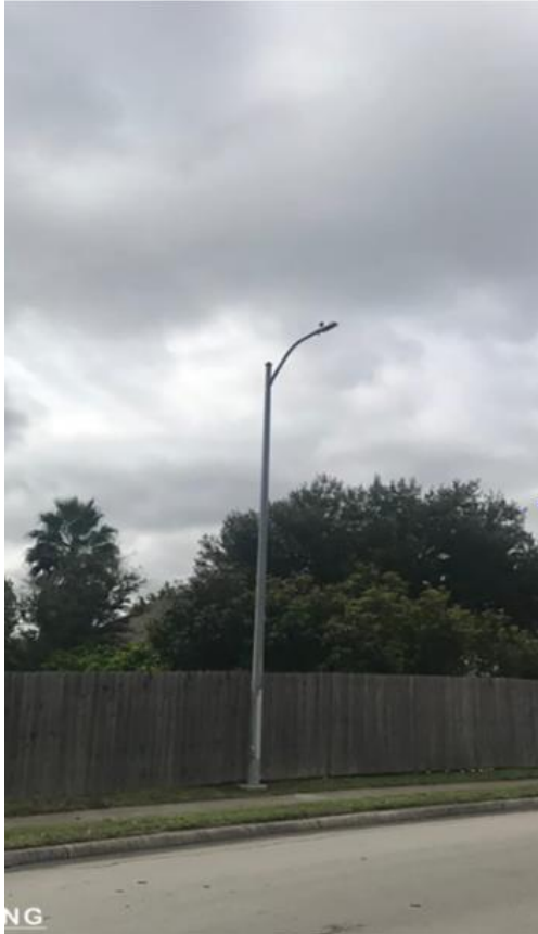
Existing CPS Energy Pole
