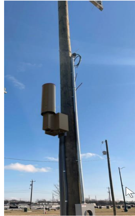
CPS Wood Pole "AFTER"
