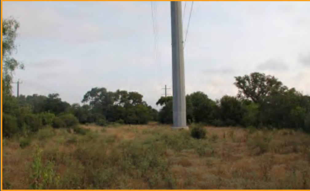
100ft clearing around transmission structure
