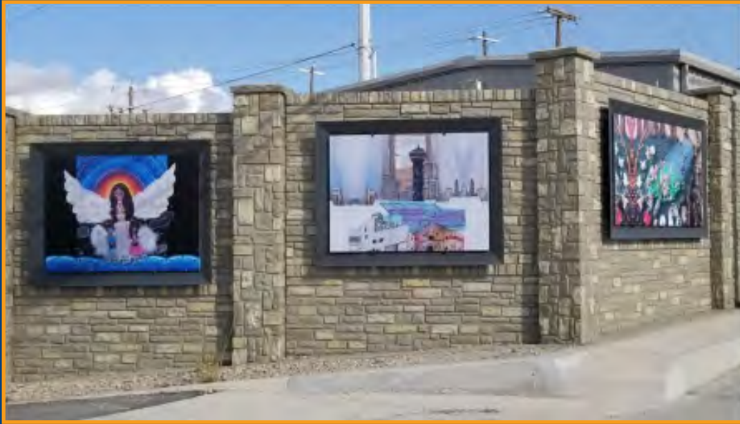
Dresden Substation – Decorative concrete wall (Art work provided by City of San Antonio)
