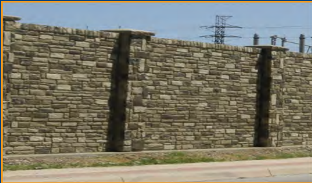
Ball Park Substation – Decorative concrete wall
