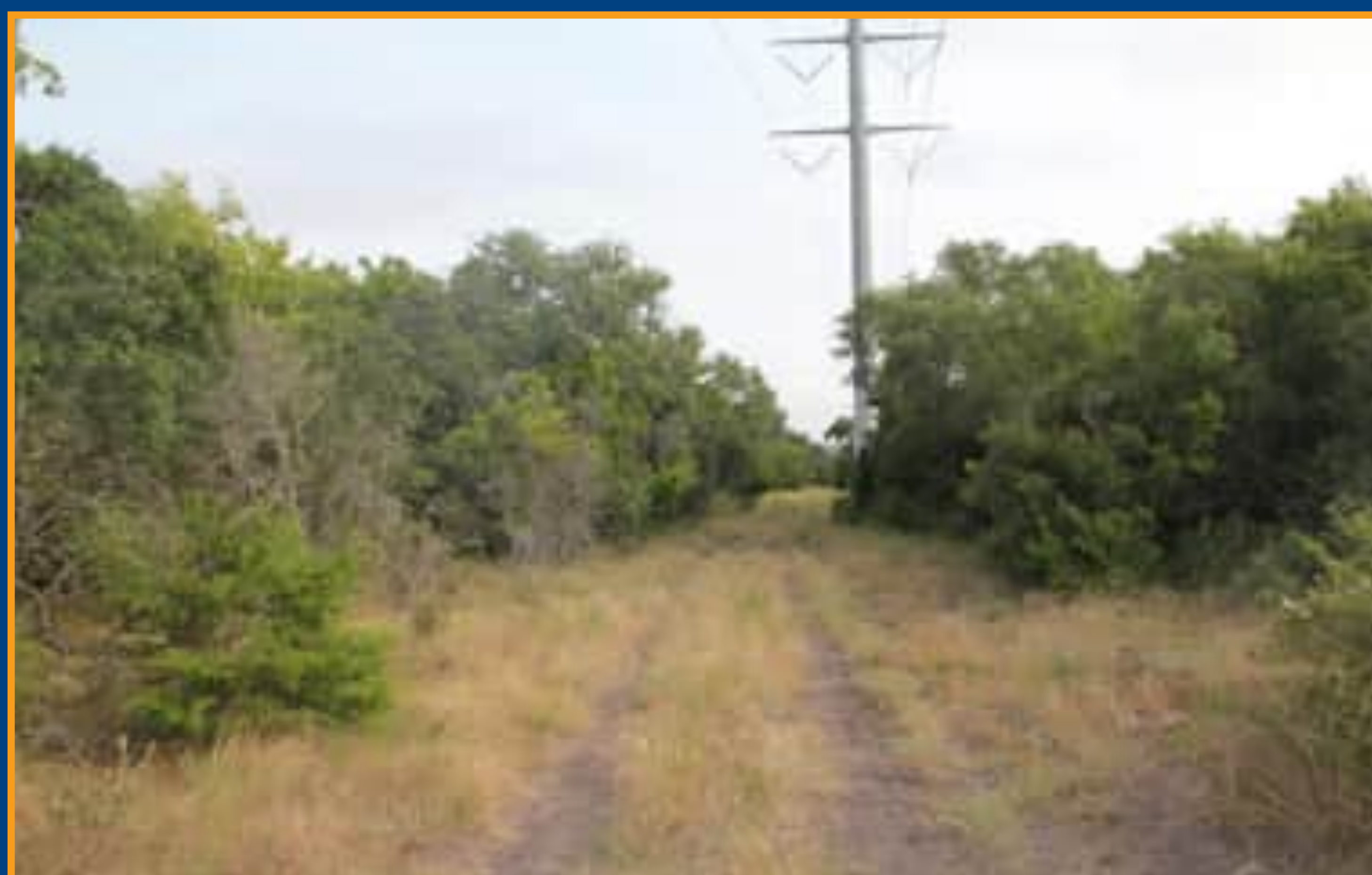
Clearing along route
