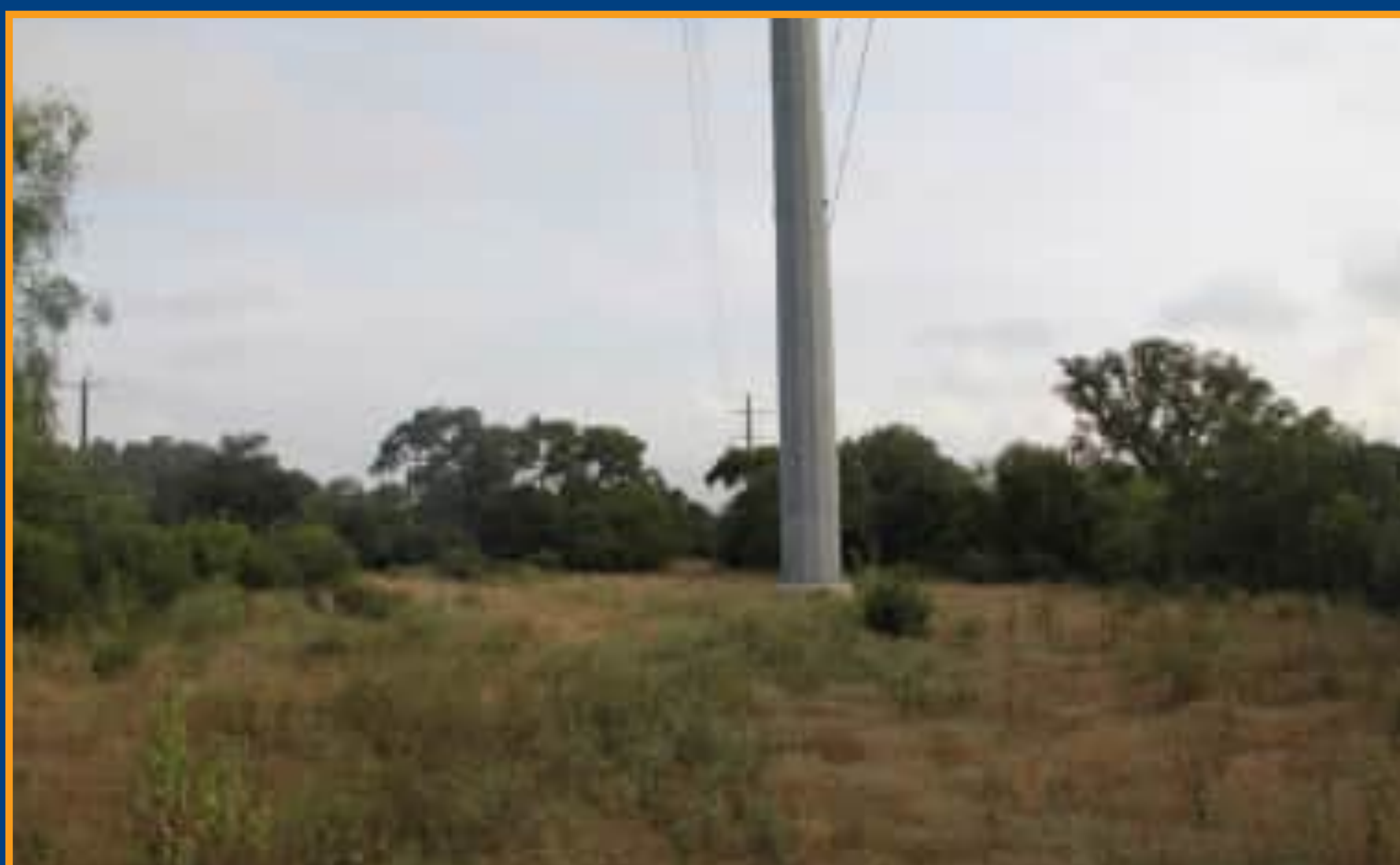
Clearing around transmission poles
