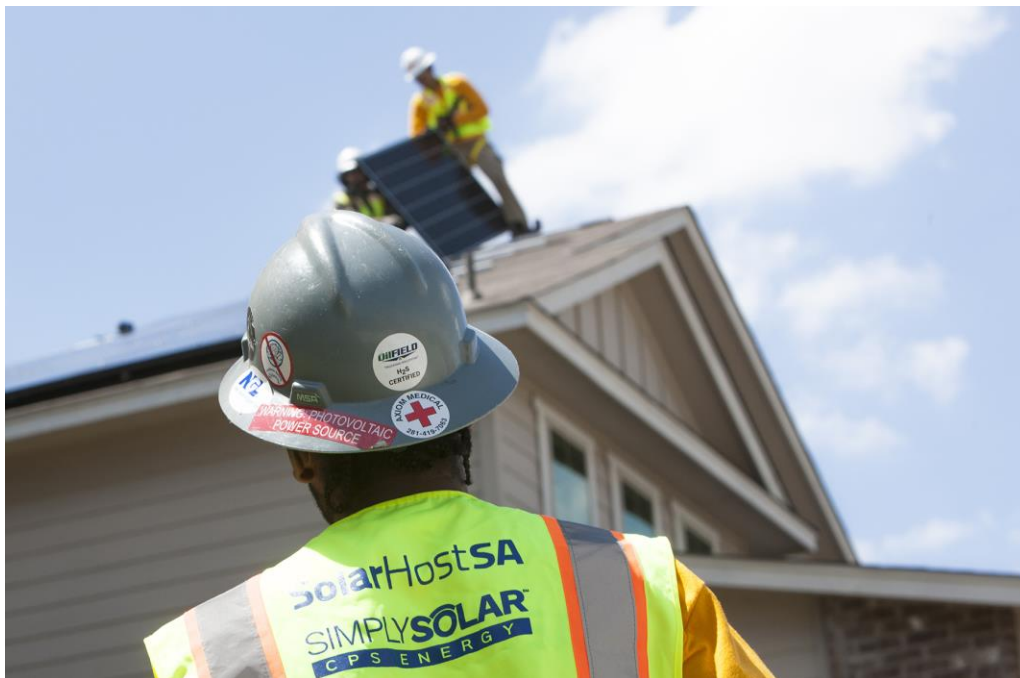
Picture 2. SolarHostSA Installation
