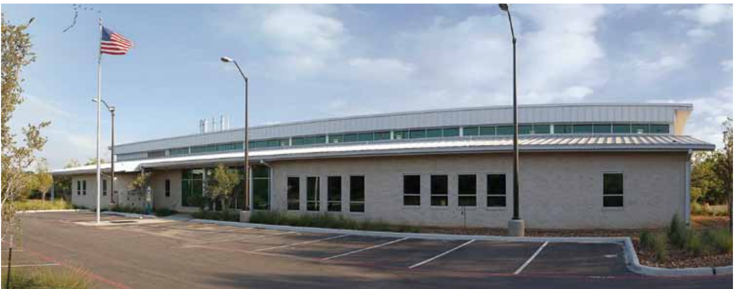
Environmental lab building at the Calaveras Power Station
