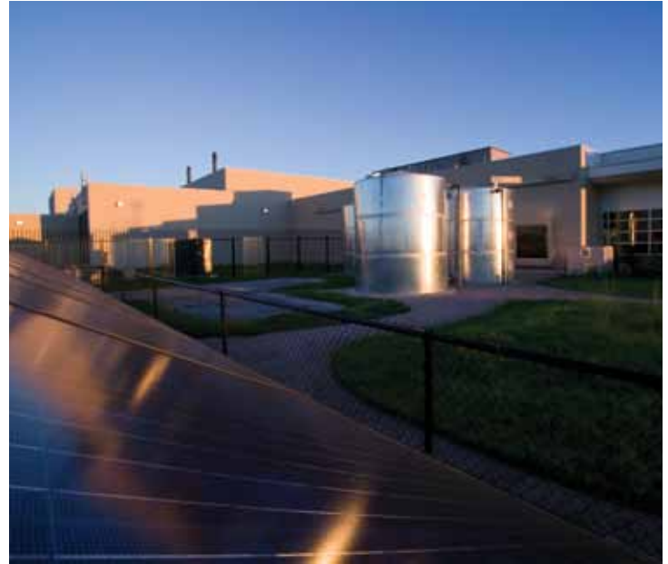
20-kilowatt photovoltaic solar panel array at the Emergency Management Center
