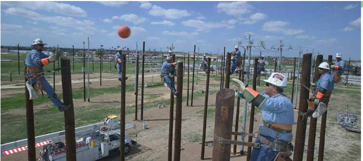
Linemen training at the Southwest Service District
