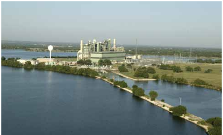
Braunig Power Station
