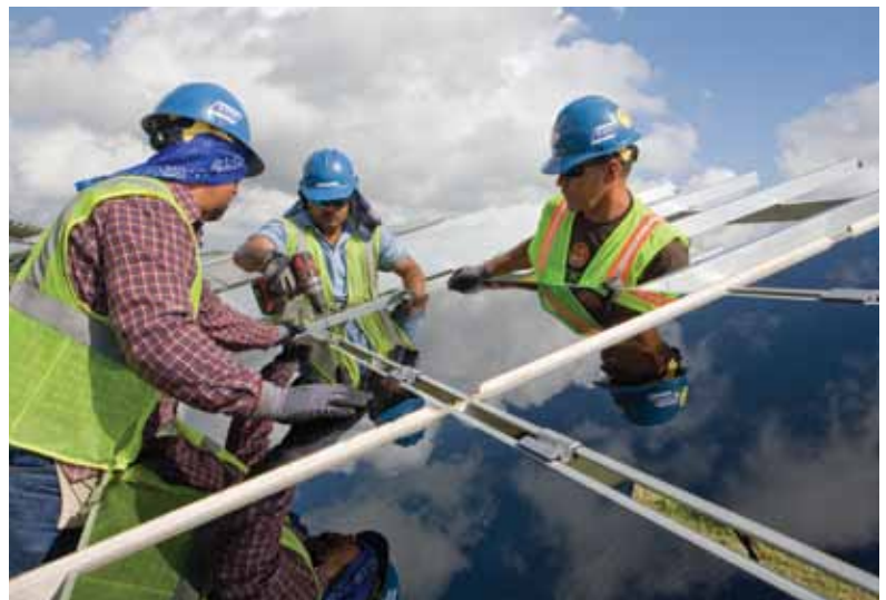
Blue Wing Solar Project under construction
