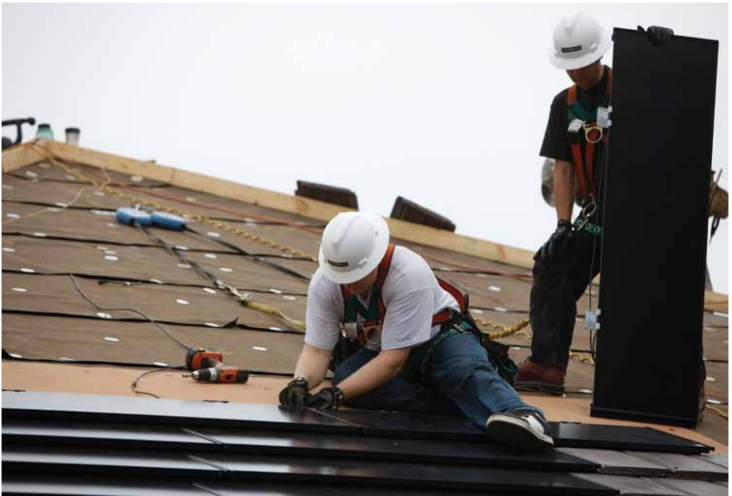
Construction on peak performance homes
