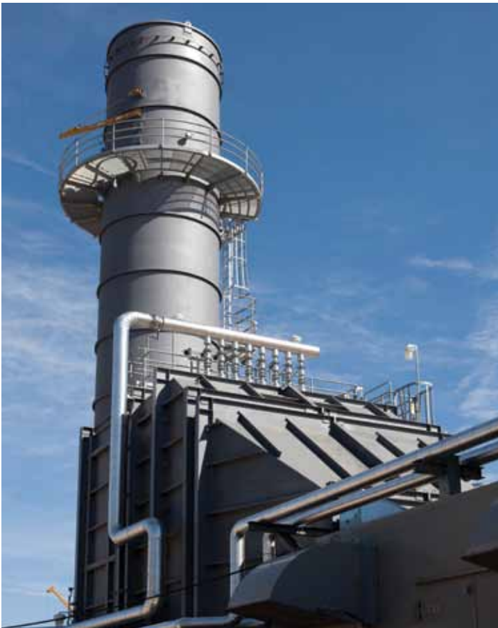
Braunig peaking units under construction
