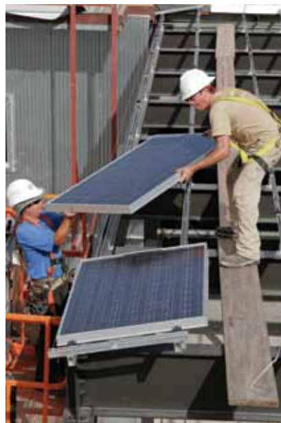
Solar panel installation at the Pearl Brewery
