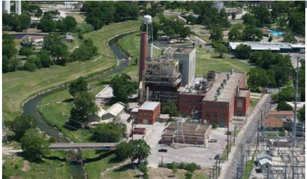
Mission Road Power Plant
