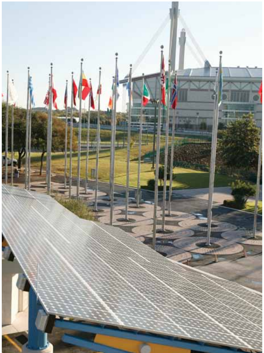
10-kilowatt photovoltaic solar panel array at the Institute of Texan Cultures
