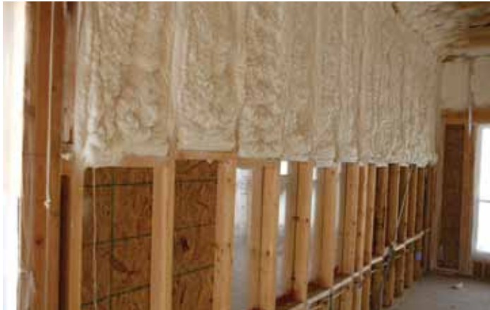
Spray foam insulation application
