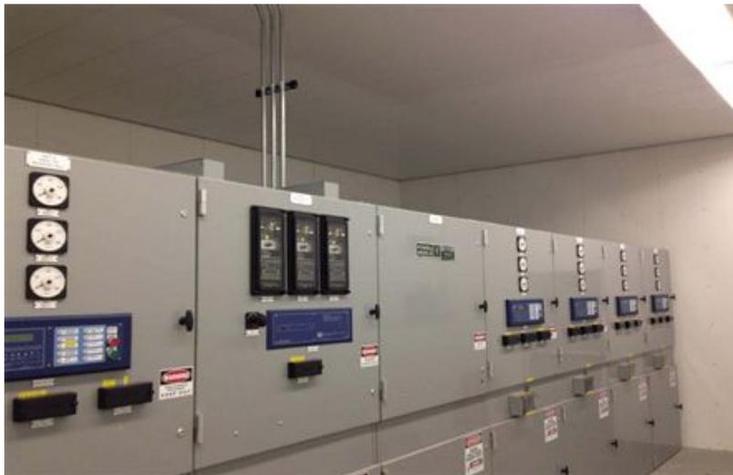
Figure 2- Internal View Substation Metal-Clad Switchgear
