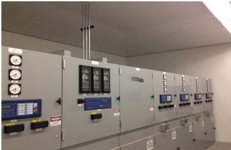
Figure 2- Internal View Substation Metal-Clad Switchgear
