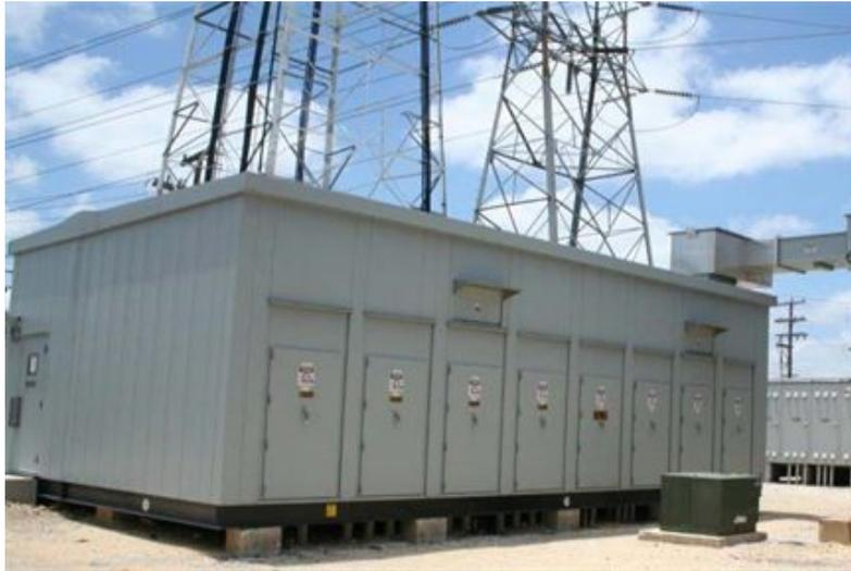
Figure 1- External View Substation Metal-Clad Switchgear
