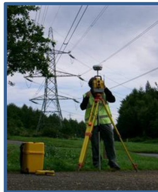
Surveying a Utility Easement
