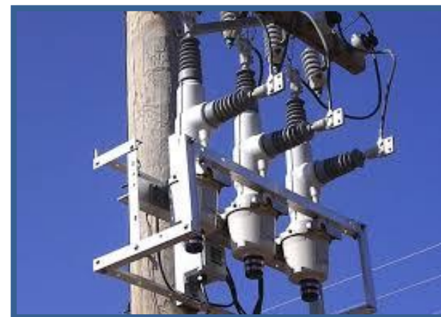
Recloser Installed On Pole
