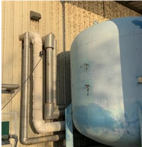
The Braunig Station 8" water processing system supply pipe did not freeze in 2011.
