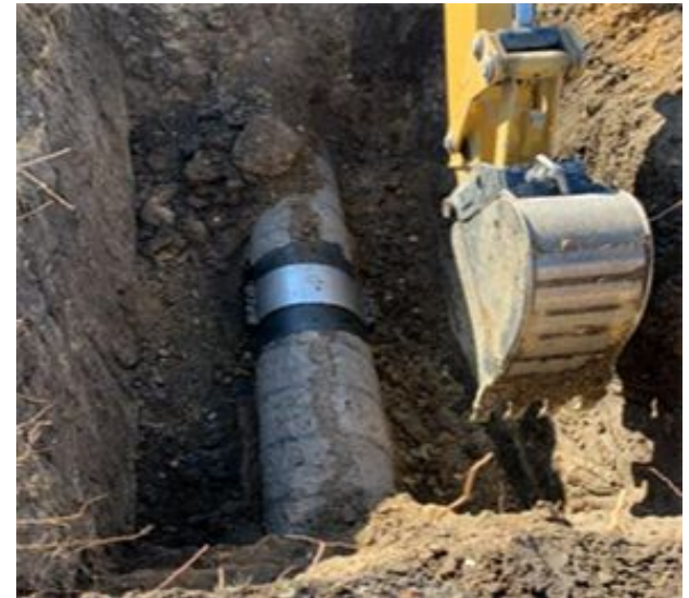
Gas Leak Repair
