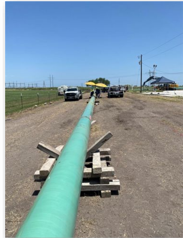
Steel Gas Main Extension
