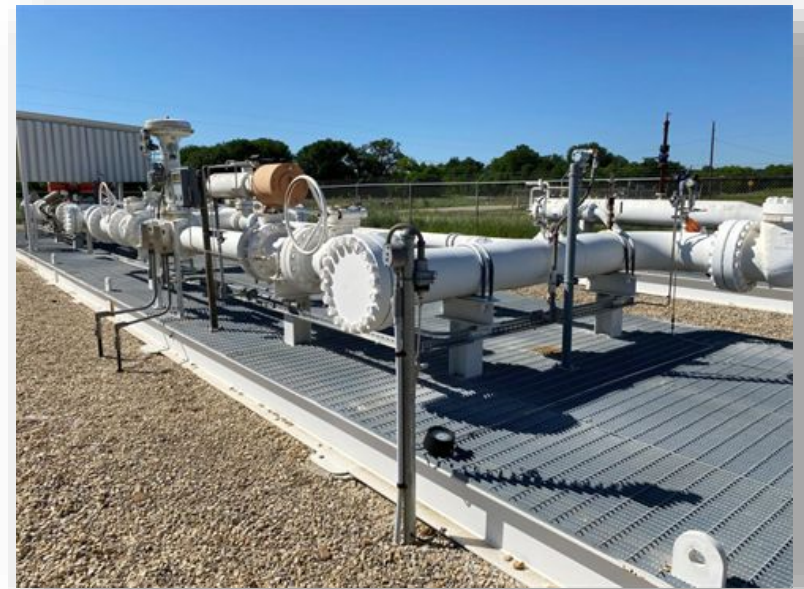
Guadalupe Transfer Station
