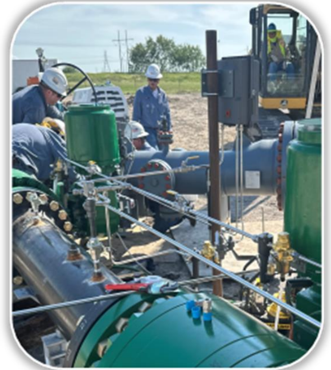
Gas Pressure Control Team performing inspection and maintenance of critical infrastructure.
