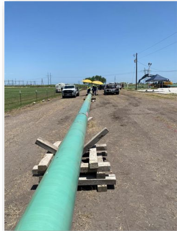
Steel Gas Main Extension
